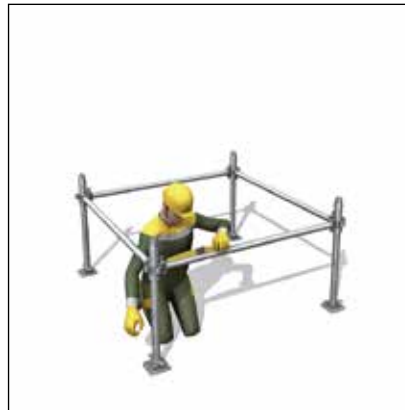
- Location and levelling.
