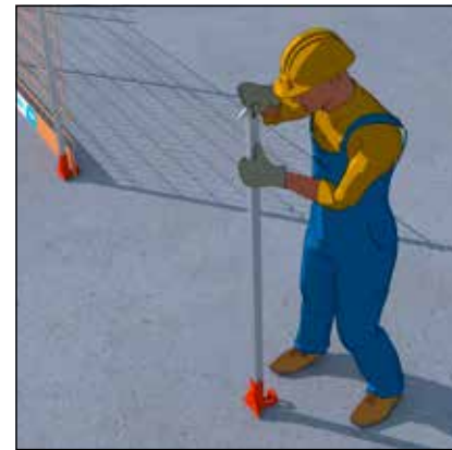
- Clip the post in the adapter.
