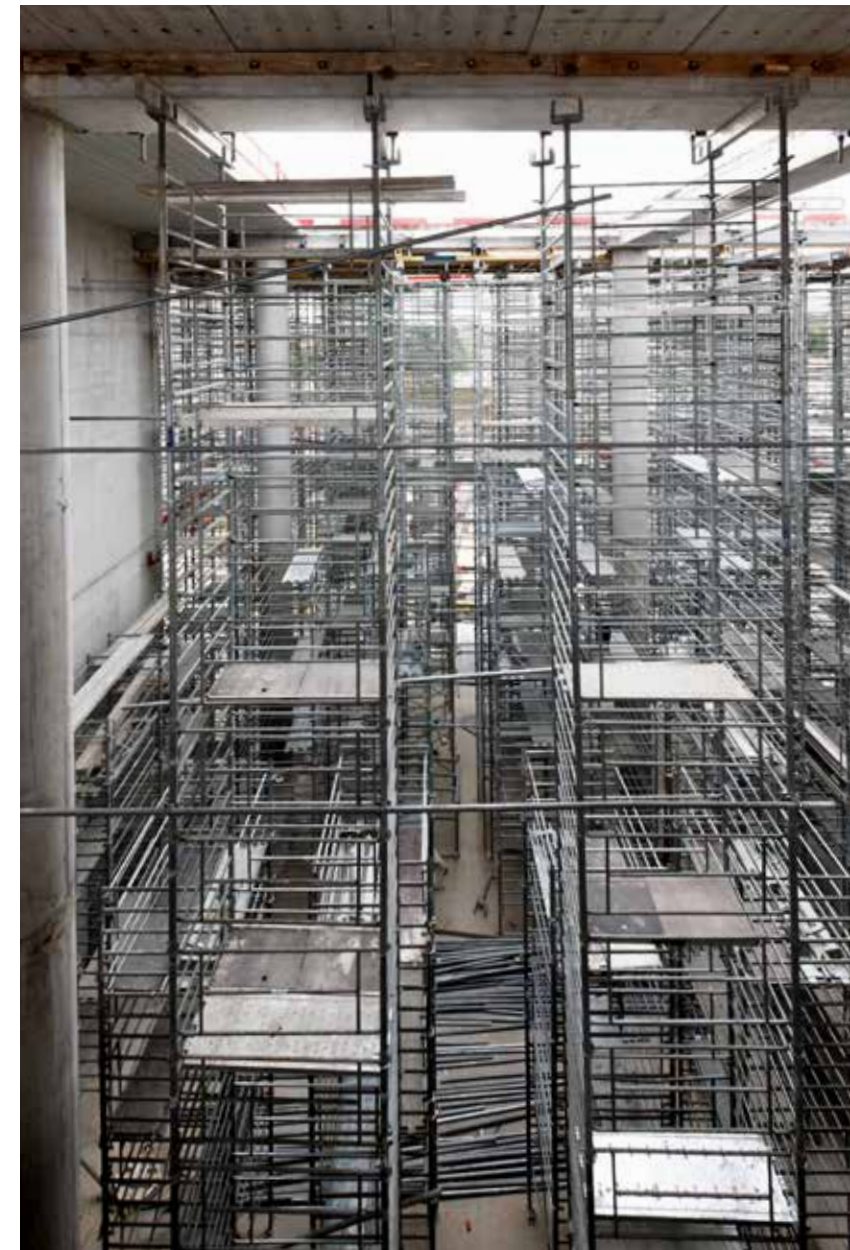
Shoring up to a height of 16 m
