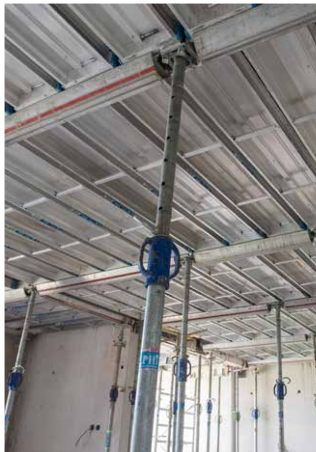
The TopDalle Eco system forms a solid surface to work in safety
