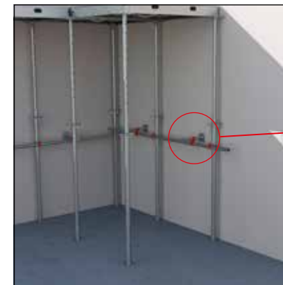
- Set up the stabilisation of the first components. - Once in place, the tripods can be removed.
