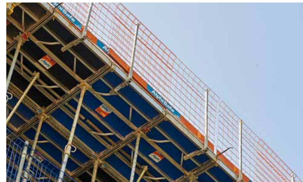
The AlphiSafe collective system allowed for completely safe installation
