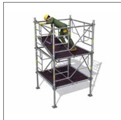
- Access to the upper level and then installation of the 2 nd plank with trapdoor.
