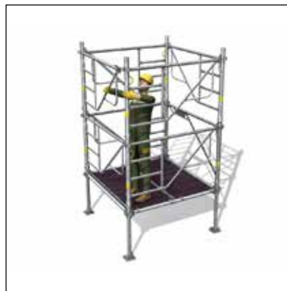
- Install two 1-m planks with trapdoor and assemble the 2 nd level.
