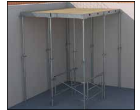
- A cross-member frame is fitted provisionally on the first 4 props.
